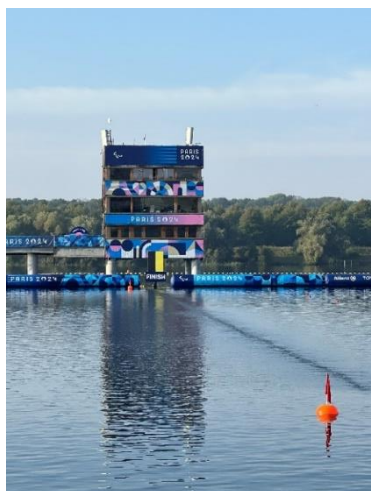
Finish Tower (判定塔)
